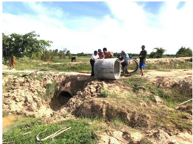
A new canal
